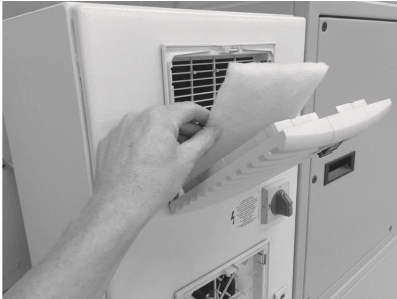
Fig. 131: Filter replacement in control cabinet
