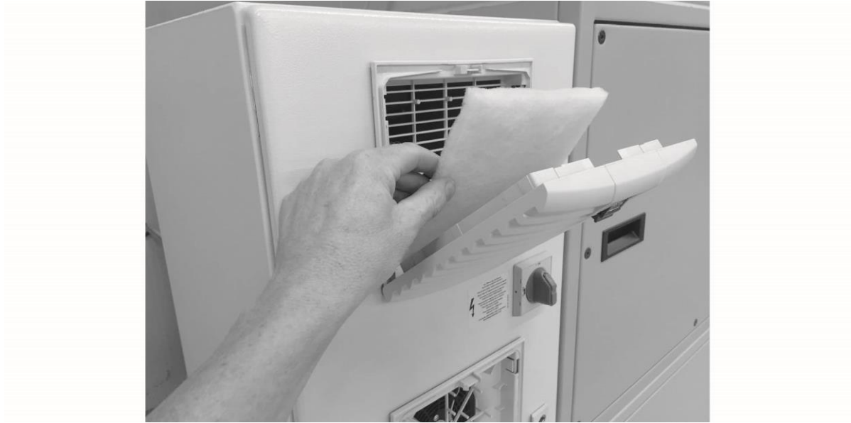
Fig. 57: Filter replacement in control cabinet
